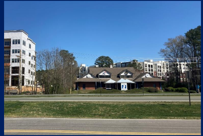
Existing development View from Fordham Blvd
