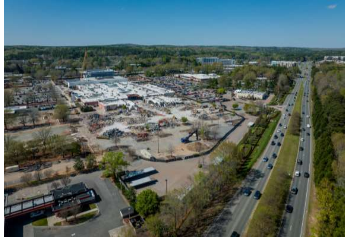
Aerial view of demolition from the southeast
