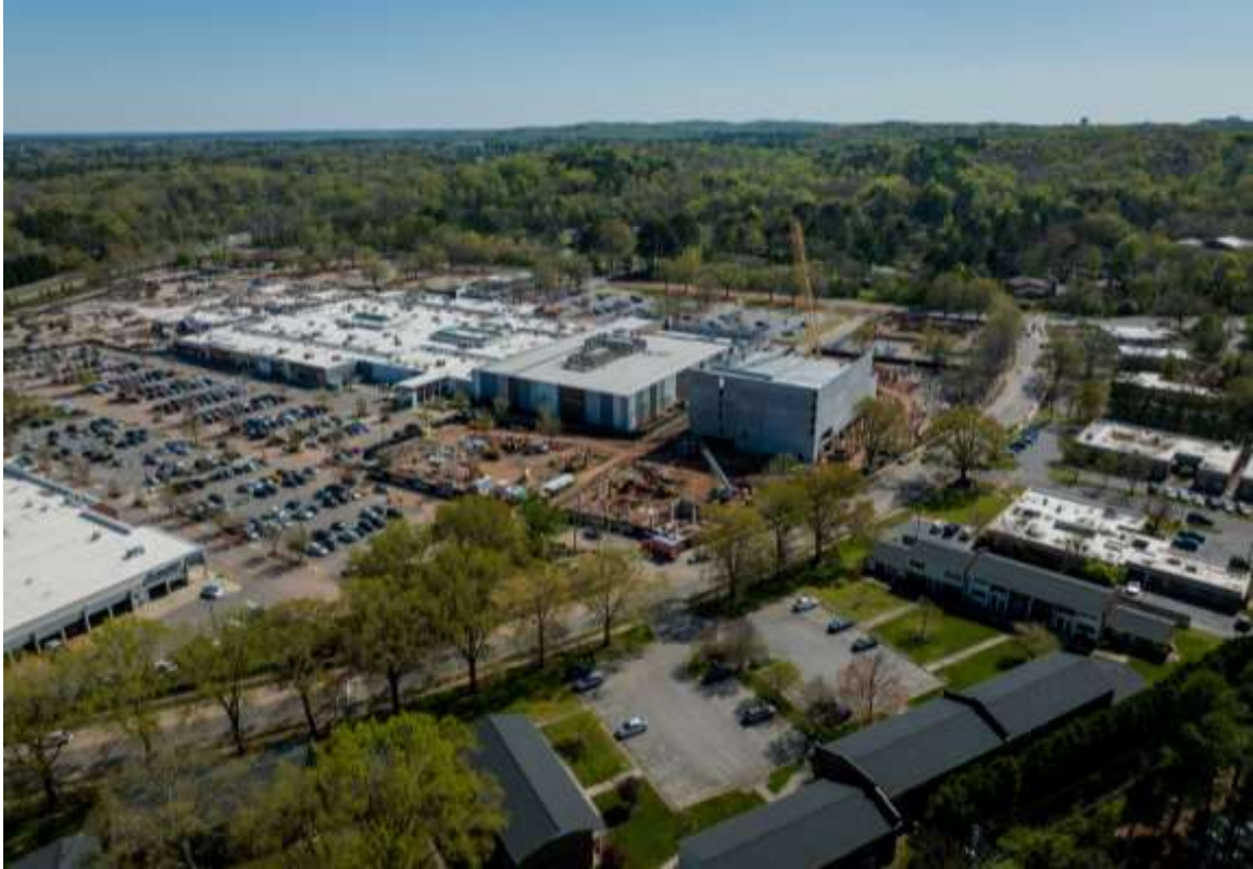
Aerial view of demolition from the northwest
