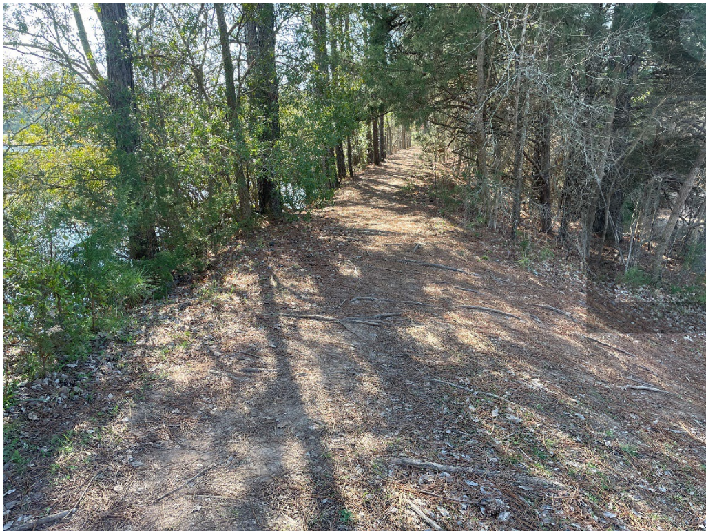
Photograph 2 – Dam Crest Facing East from West Abutment
