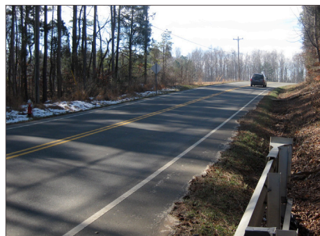
Homestead Rd. at grade.
