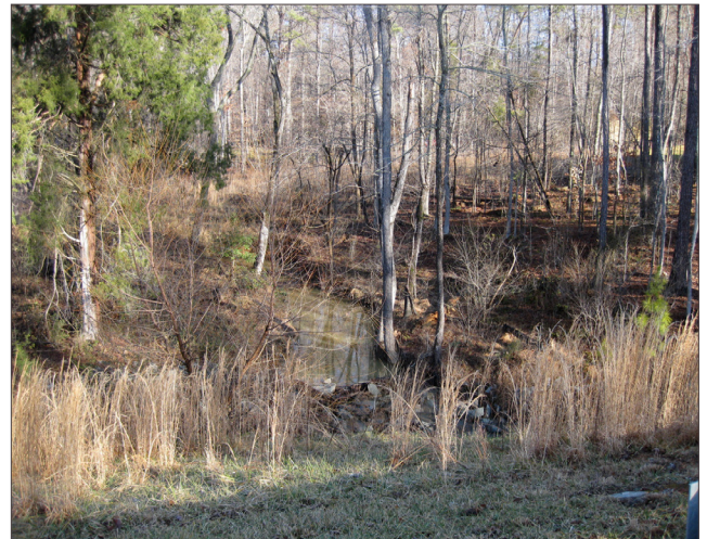
Creek crossing conditions beneath Turtleback Crossing.
