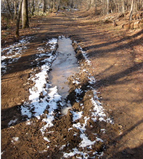
Maintenance vehicles and overuse have contributed to erosion along the corridor.
