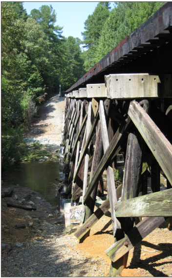
Railroad overpass at Estes Dr.
