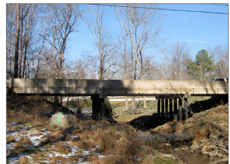
Bridge at Homestead Rd.
