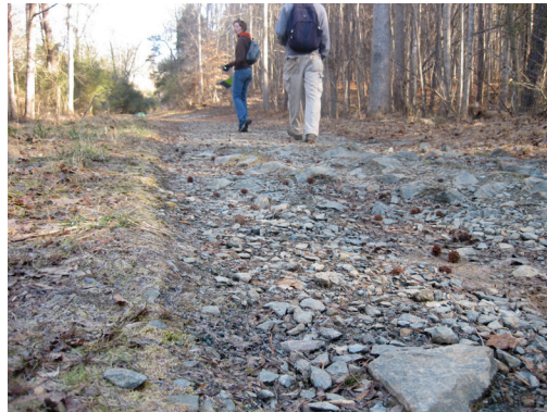
Hardscape materials imported onsite have furthered erosion problems.
