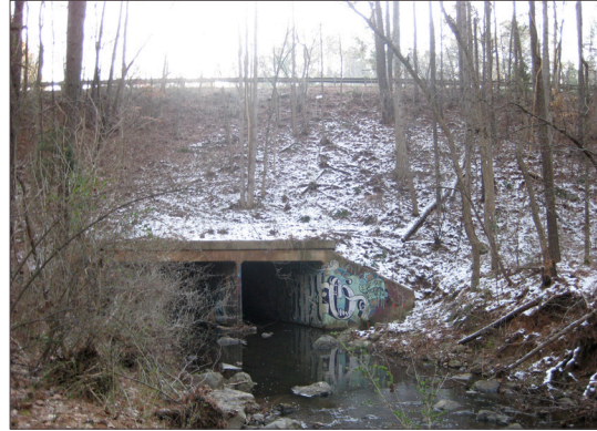
The box culvert beneath Estes Dr. extension.
